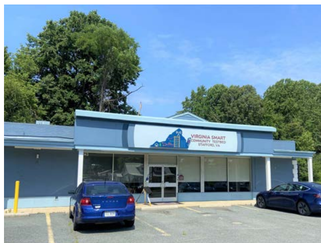
STAFFORD - BUDOVA SMART COMMUNITY TESTBED
